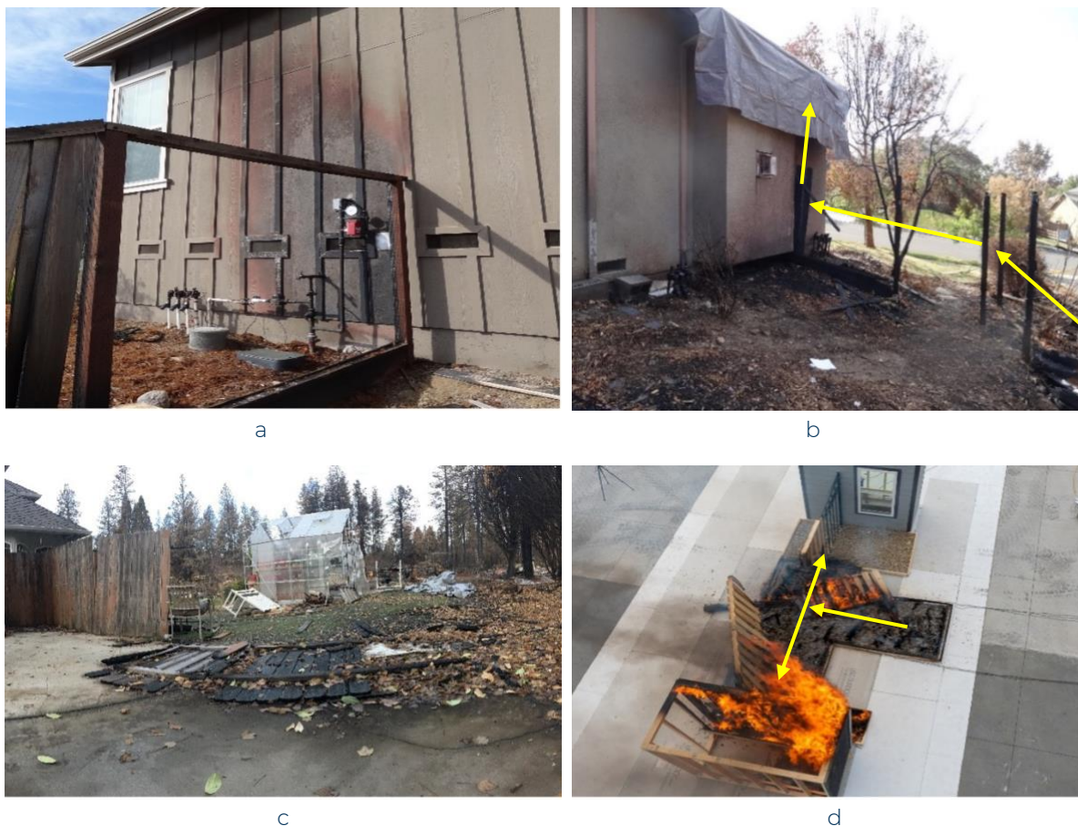
Figure 6. Examples of combustible fencing providing a pathway for fire to the house, damaging the noncombustible siding and eave (a and b) in the Glass Fire (2020) in Napa and Sonoma Counties, California, defended; (c) in the Camp Fire (2018) in Butte County, California, defended by first responders ( Insurance Institute for Business & Home Safety, 2020 ); and (d) at the IBHS Research Center where the arrows indicate the direction of fire spread.
